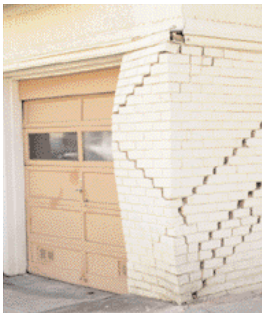
Figure 4.44 Even if the ground beneath a building was uniform when the building was constructed, shear damage can occur. An earthquake caused this damage.
